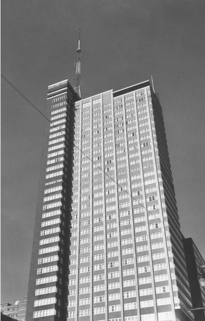
Rooftops of skyscrapers offer breathtaking views as well as being excellent locations for broadcaster's antennas. This building is in Philadelphia. ( Kyle Kirkland )
