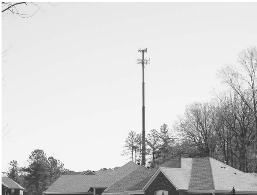
In August 2005, Hurricane Katrina damaged this cell phone tower in Clinton, Mississippi, leaving residents in the neighborhood with unreliable cell phone service until repairs were made. ( Kyle Kirkland )
